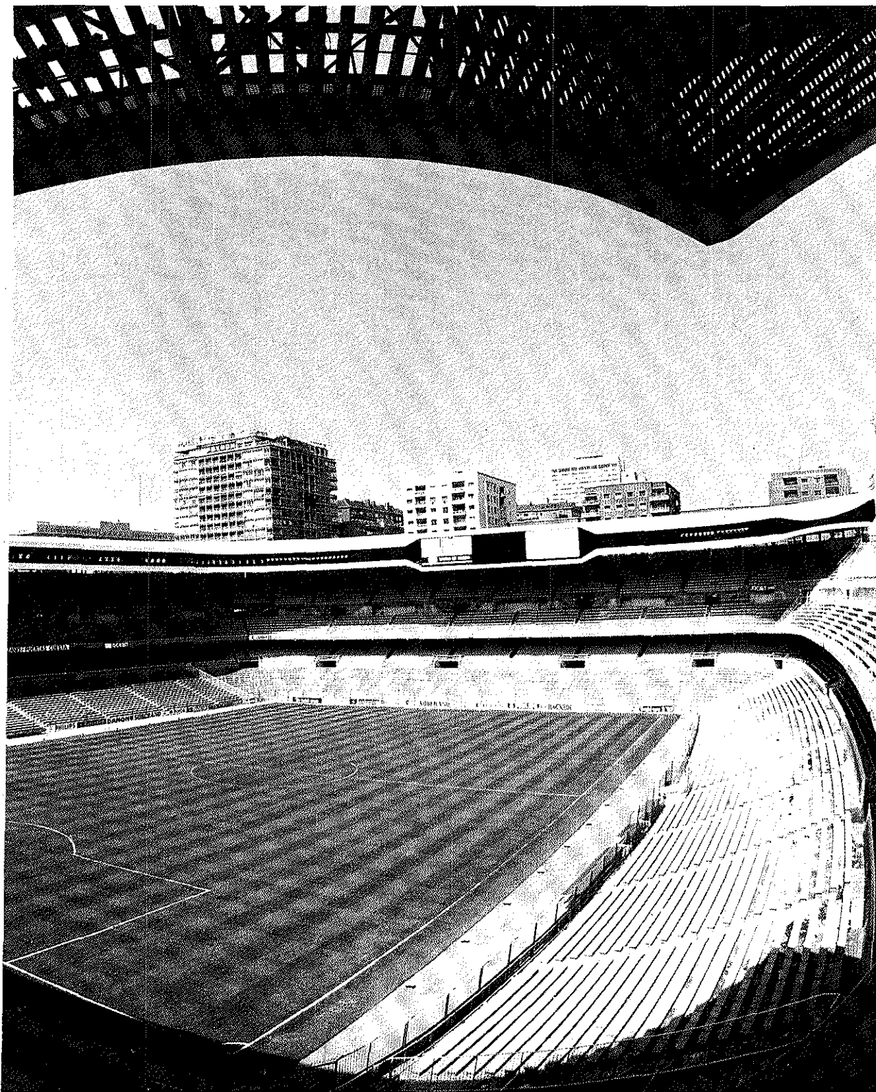
Lightweight concrete components reinforced with Cem-Fil alkali-resistant glass fibres have been used extensively at the Real Madrid football stadium.
